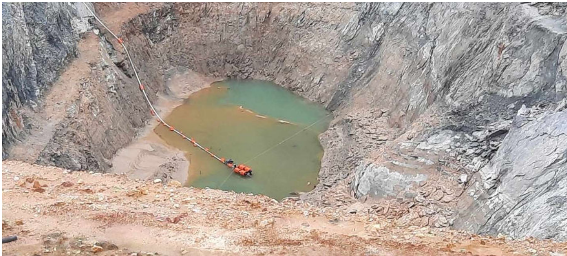
Figure 3: Cannon open pit dewatering progress, September 2024.
