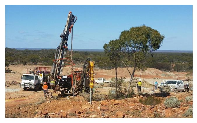
Figure 3: Commencement of grade control drilling in the Regal area of Boorara
