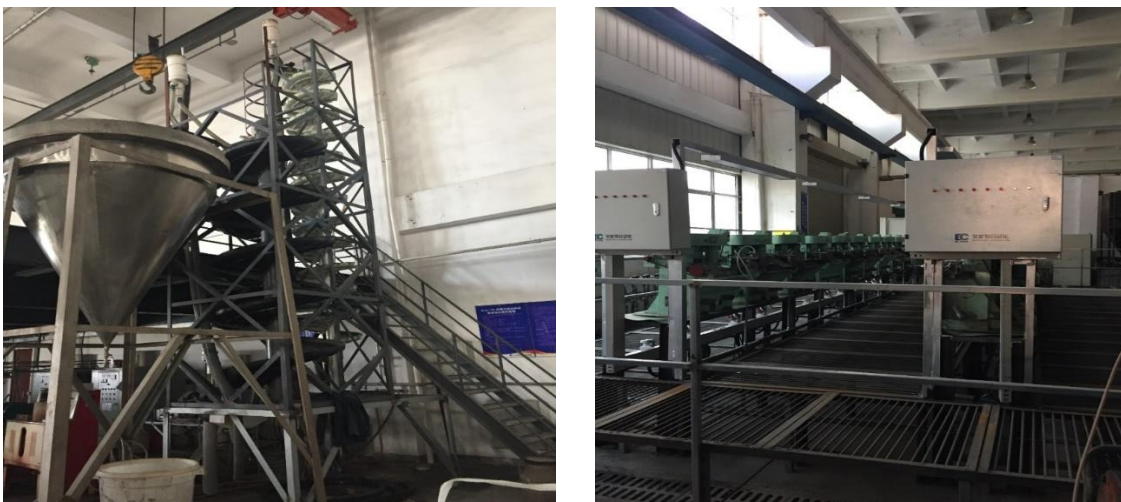
Figure 11: Hunan Research Facility spiral and flotation circuits
